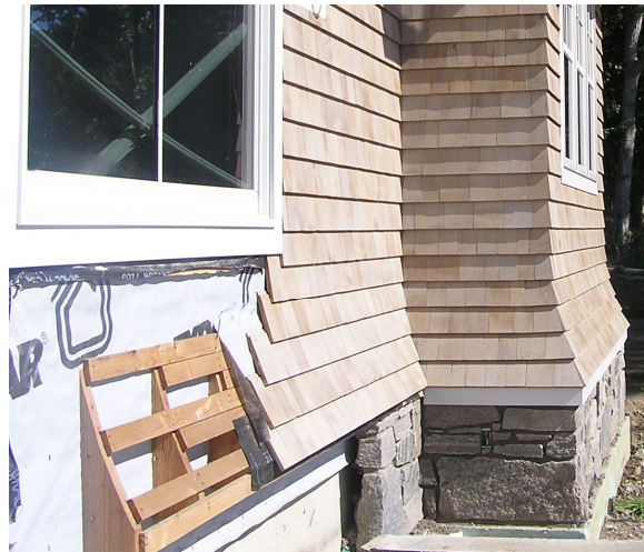
Picture of 5.5" Radius flare with additional horizontal framing and fascia trim.
