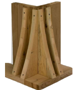
Curved Blocking at Corner
